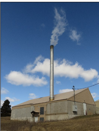
Heating plant & chip storage building.
