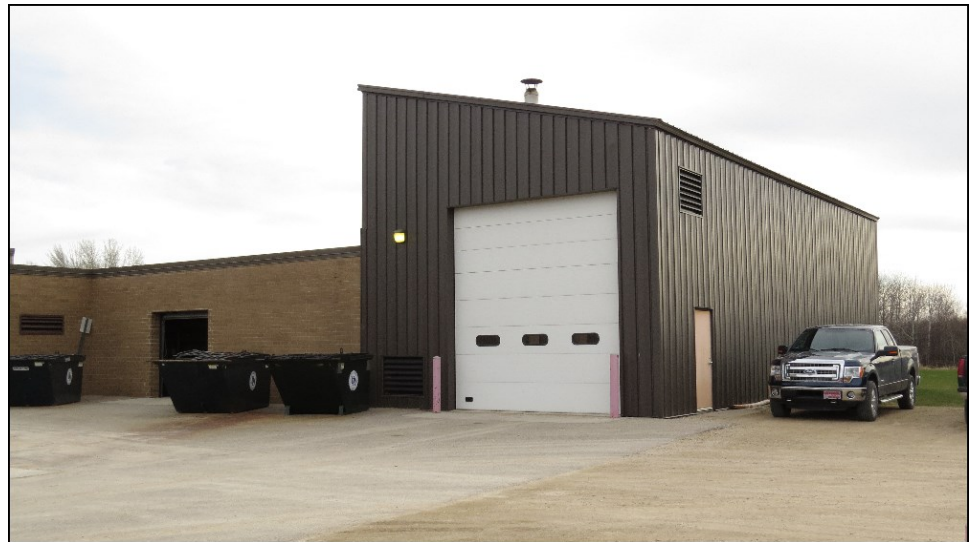
Heating plant building with drive-in bay for wood chip delivery.
