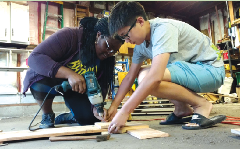
Hanbing Liang (right) and Stephanie Onwenu (left) constructing window shutters.
