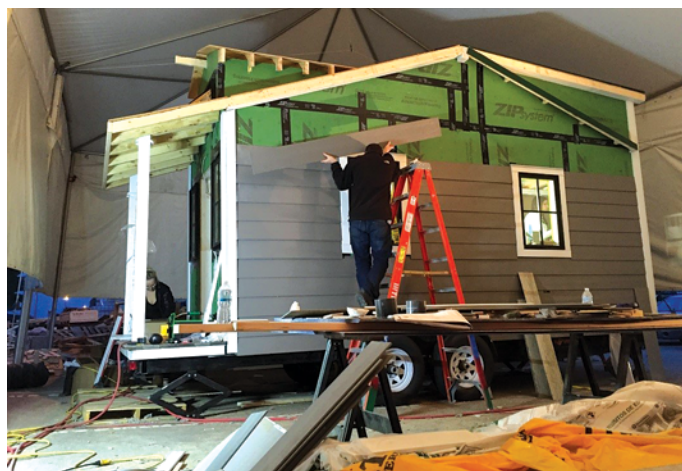
In true LA fashion, an all-night work crew to get the interior and exterior wall coverings installed for the ribbon cutting.
