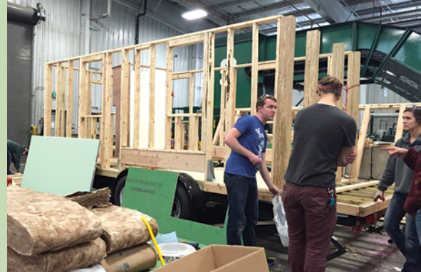
Walls going up with Tom Lyons leading the front porch installation.
