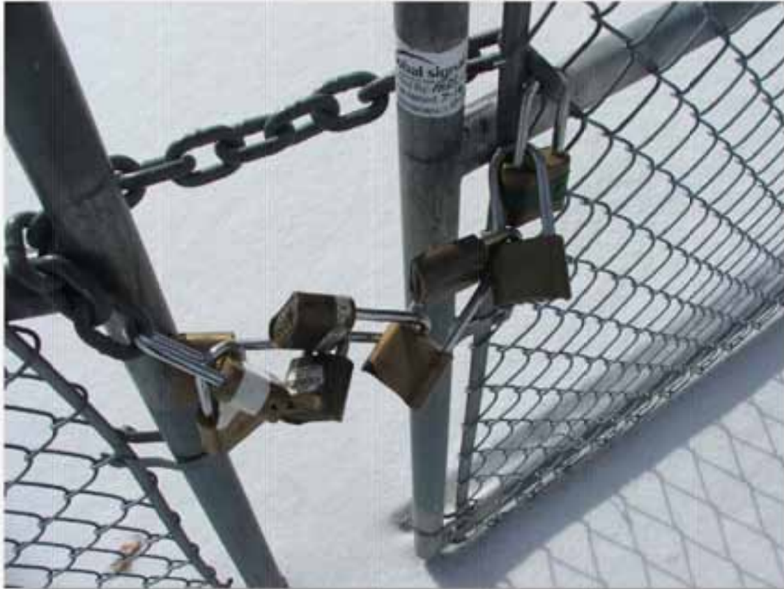
Figure 30: A Variety of Locks from Each Service Provider bar the Entrance to a Co-location Tower Compact Area in Lansing.
