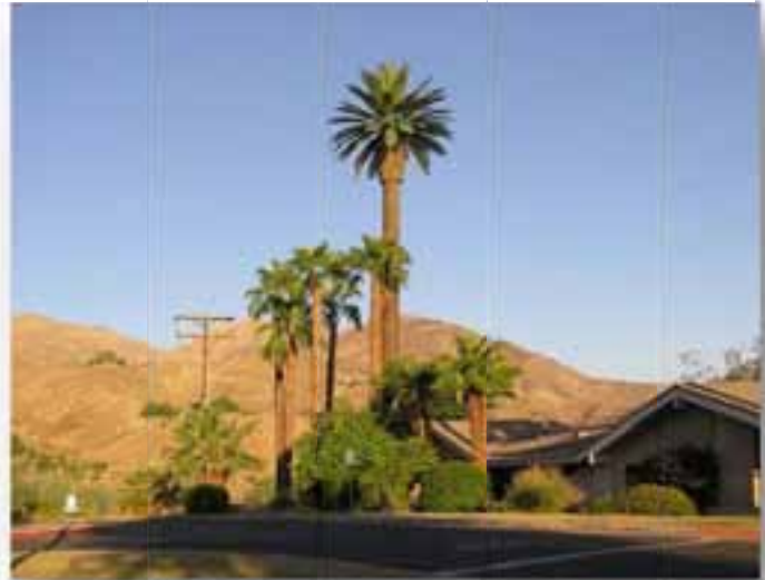
Figure 23: A Monopalm with Hidden Antennas located in Palm Desert, California Source: (Kramer, 2007)
