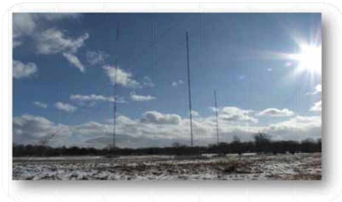
Figure 18: Guyed Towers located at 600 W. Cavanaugh Rd. The Towers are 62.5 feet above ground-level, and are owned and managed by MAC Donald Broadcasting Company.
