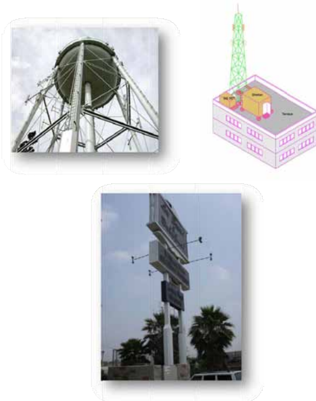
Figure 14: A Tank Mount, Rooftop Tower, and Signage Tower
