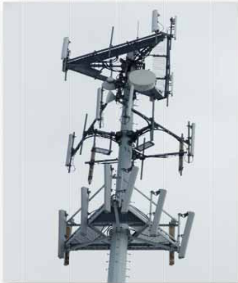
Figure 31: Co-location Antennas on a Monopole Tower located at 3128 South Martin Luther King Boulevard in Lansing, Michigan.
