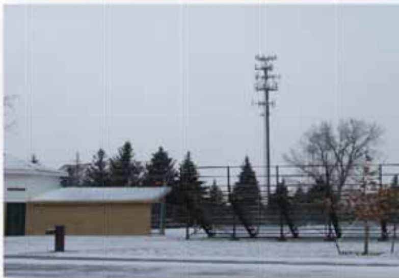
Figure 15: A Monopole Tower located at 125 South Clippert St. The Tower is 60.7 feet at ground-level, and is owned and managed by AAT Communications Corporation.
