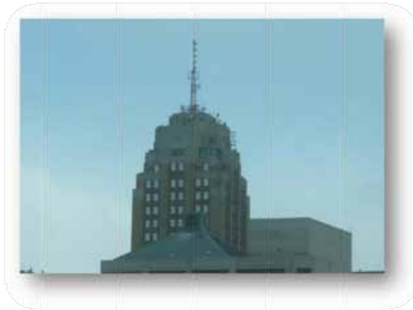
Figure 17: A Rooftop Lattice Tower located at 530 W. Allegan St. The Tower is 100 feet above ground-level, and is owned and managed by SBA Communications.
