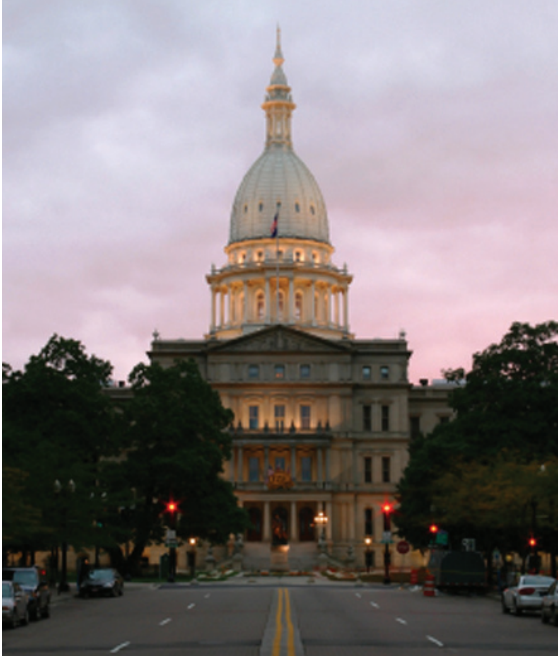
The Michigan State Capitol building in Lansing.
