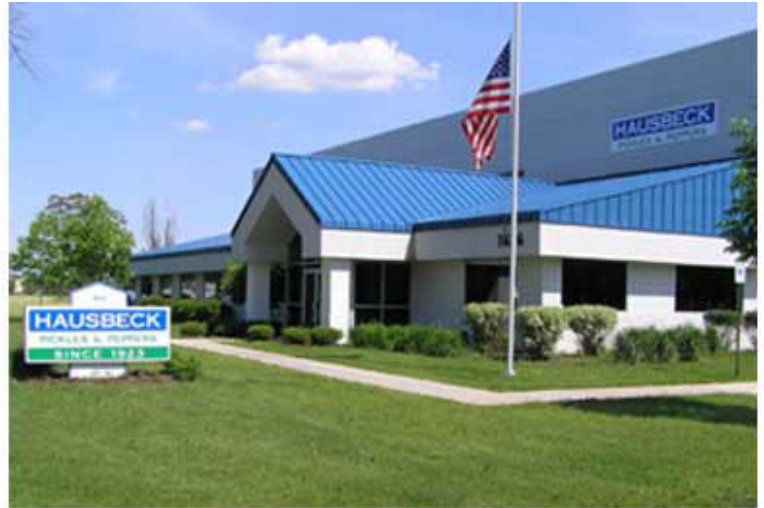
Hausbeck Pickle Company's new headquarters, warehouse space and future processing site.
