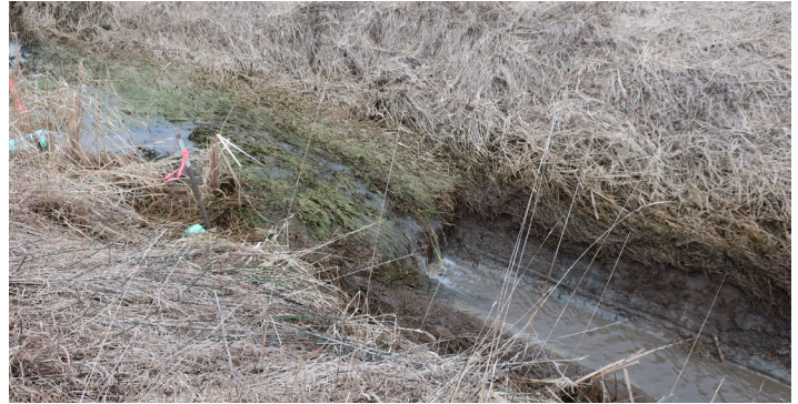
Figure 1- Top: The outlet is submerged because it is too close to the ditch bottom. Bottom: The same ditch during the process of being cleaned and deepened to allow free flow from the outlet (photo credit: Jason R. Piwarski).
