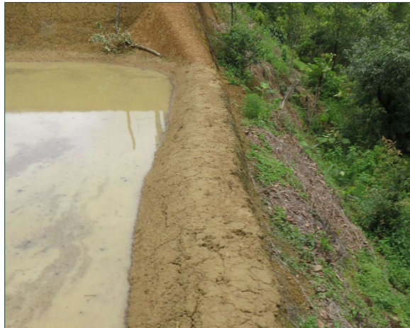
Figure 3-15. Bunds or earthen dams prepared by ramping or pressing down and plastering.
