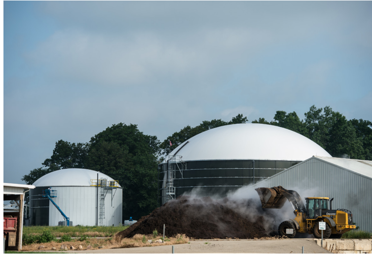
The MSU South Campus Anaerobic Digester will utilize about 17,000 tons of organic waste to generate 2.8 million kilowatt hours of electricity per year. Photo provided courtesy of the MSU Office of Communications and Brand Strategy.
